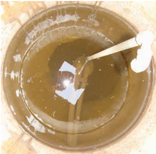
A drilled well located in a well pit (these are not to be newly constructed anymore) can be contaminated when the pit is exposed to surface water (that comes through the casing or through gaps in the cap). These wells can be upgraded to have a pit-less adapter that makes the well more secure and less likely to be contaminated. You can see evidence of water entering the well around the concrete casing joints. New construction wells cannot be located in well pits. NEVER ENTER A PIT.
