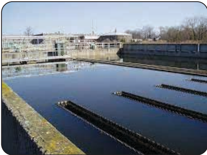
Corbett Water Pollution Control Plant
