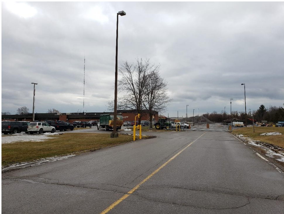
Photo 2 - Durham Works Department on the Site
