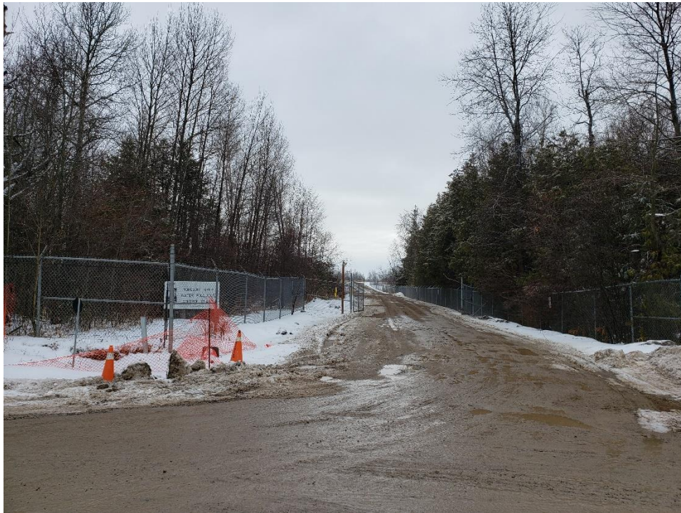
Photo 4 - Entrance to the Site on Scugog Line 8.
