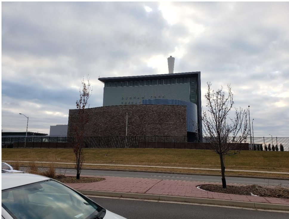
Photo 2 - Durham York Energy Centre east of the Site
