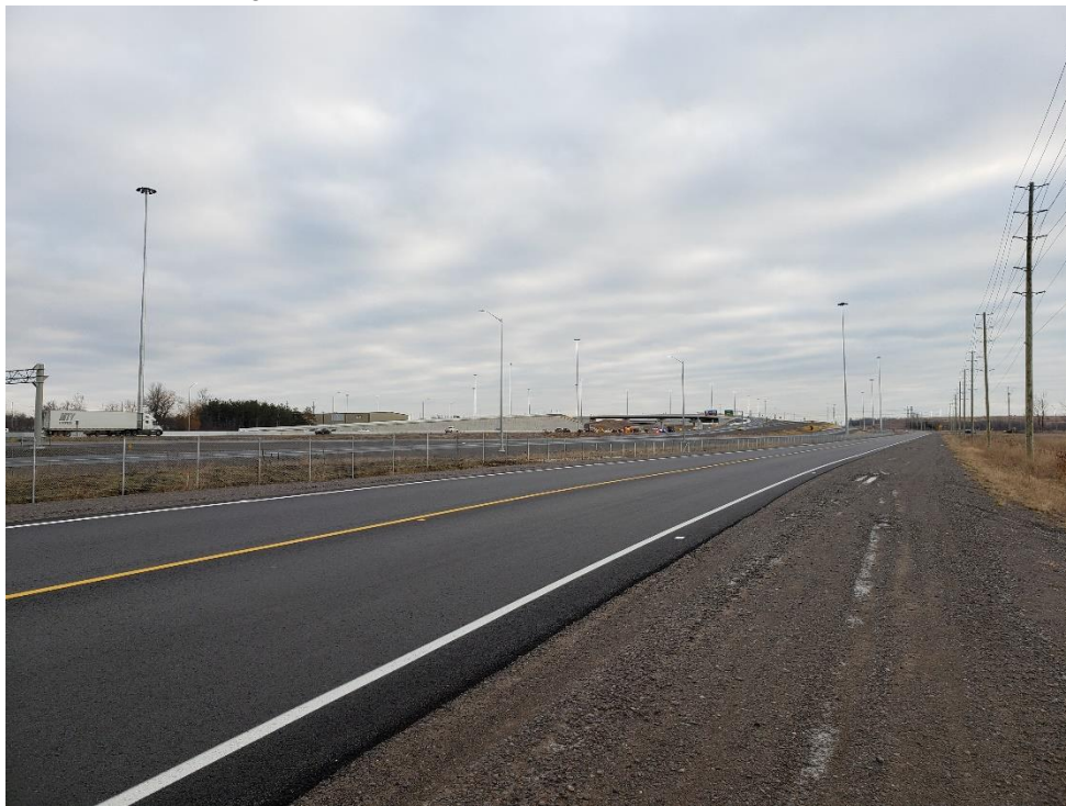
Photo 6 - New Highway 401 and Highway 418 interchange.
