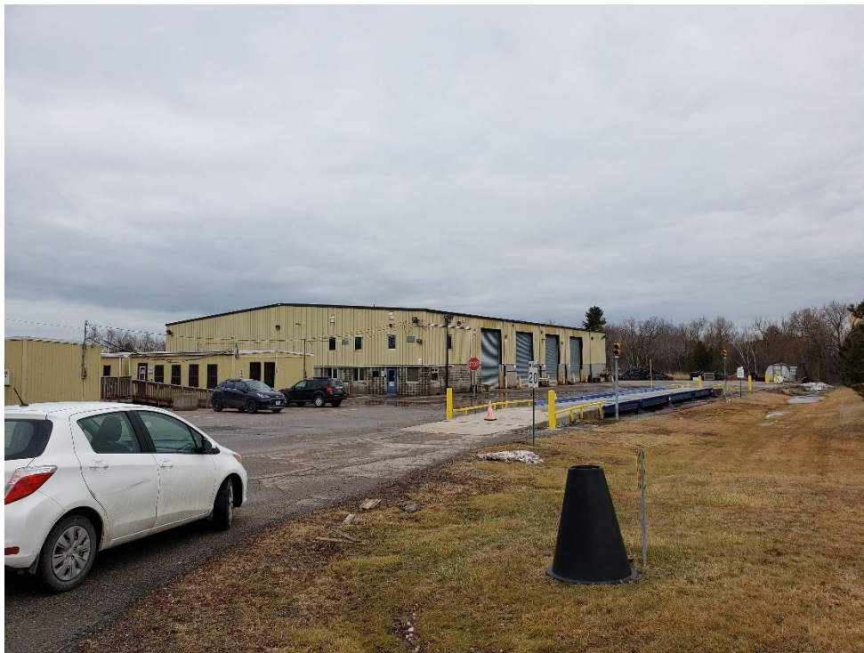
Photo 10 - South west view of the Site from end of service road.
