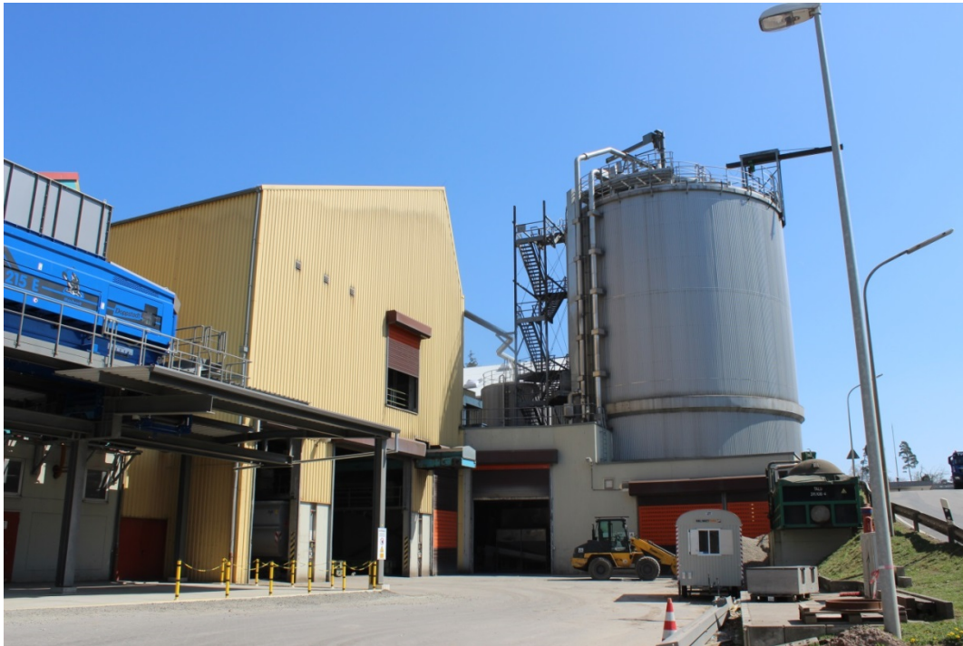
Figure 3-4-1 Anaergia, OREX, Kaiserslautern: Pre-processing Building and Digester
