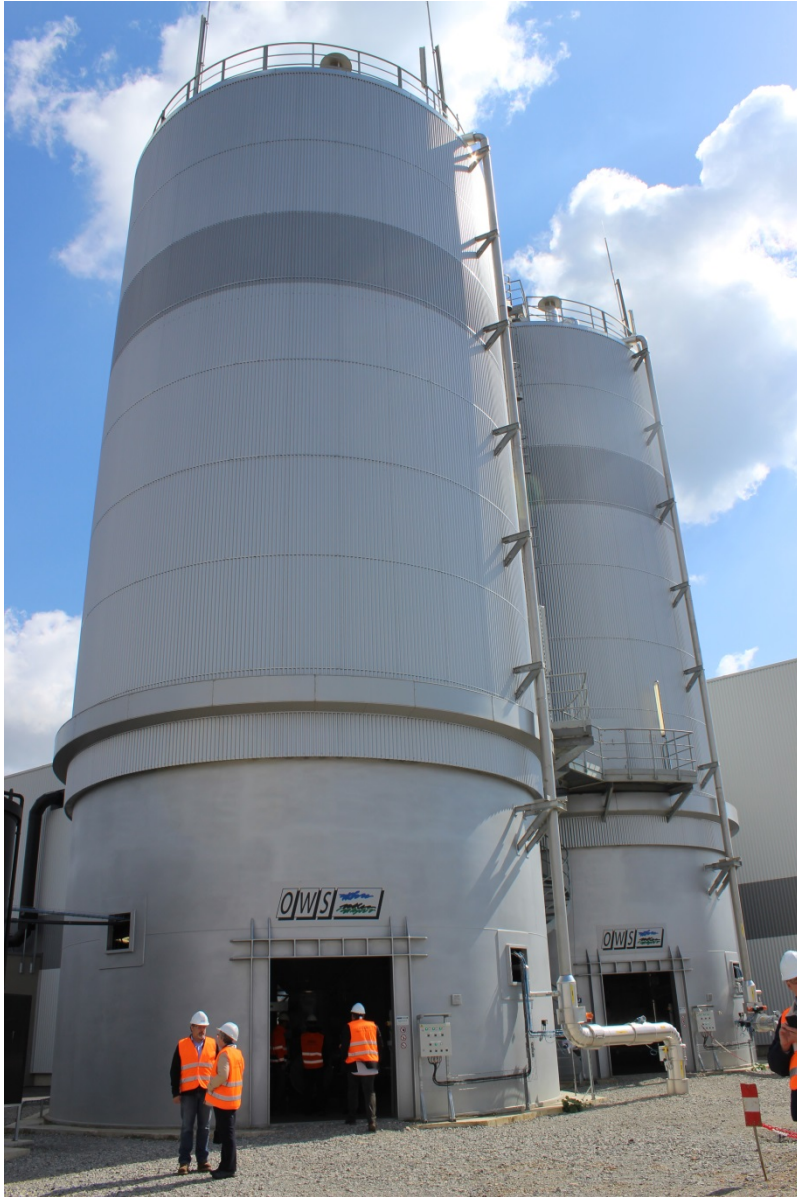
Figure 3-7-6 OWS Chagny AD Plant: AD Digesters
