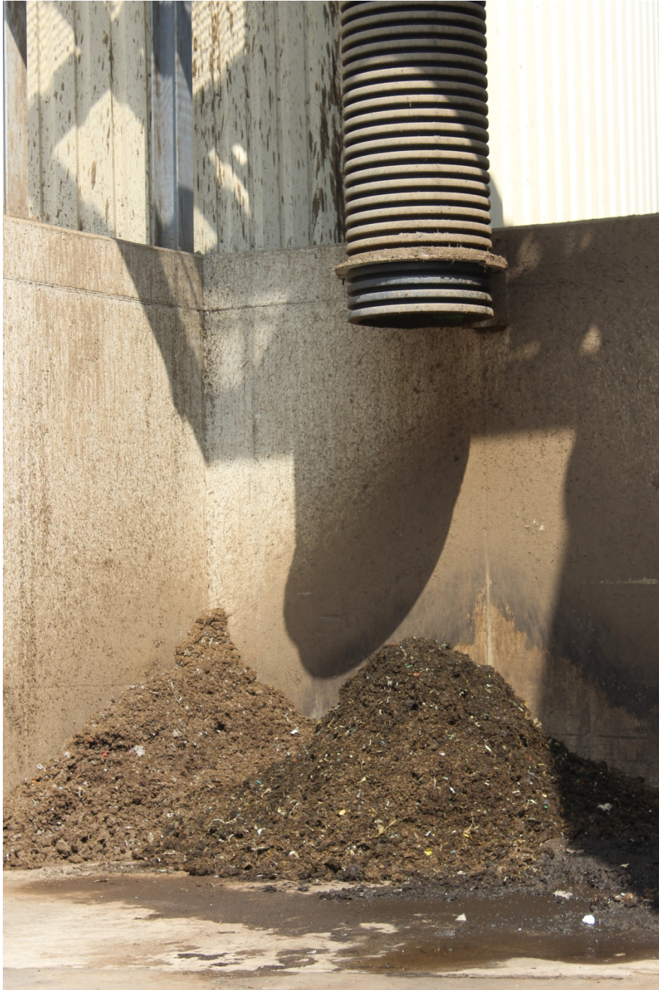
Figure 3-3-6 FITEC, Rothmuhle Biogas Plant: Light and Heavy Fractions Removed from Digester
