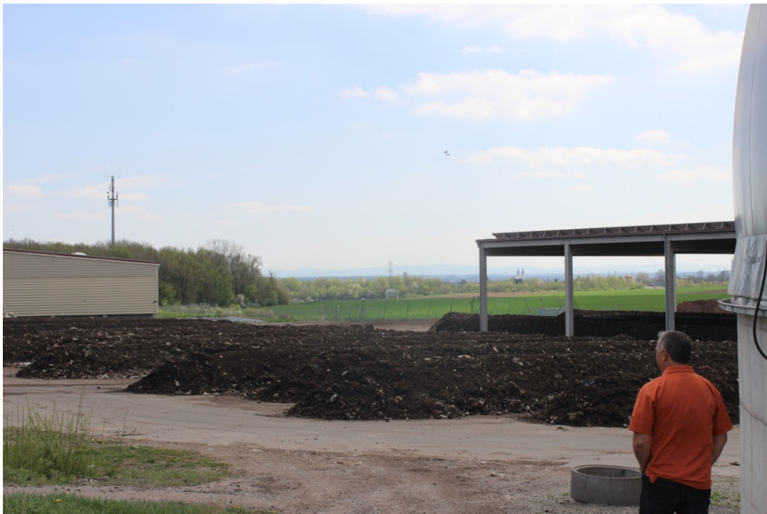
Figure 3-3-5 FITEC, Rothmuhle Biogas Plant: Composting Area
