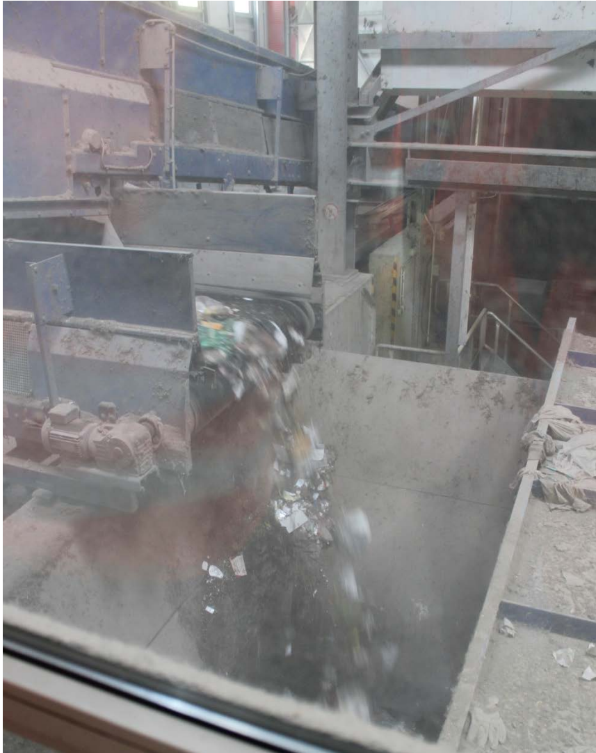
Figure 3-4-3 Anaergia, OREX, Kaiserslautern: Incoming Material Feed to OREX Hopper
