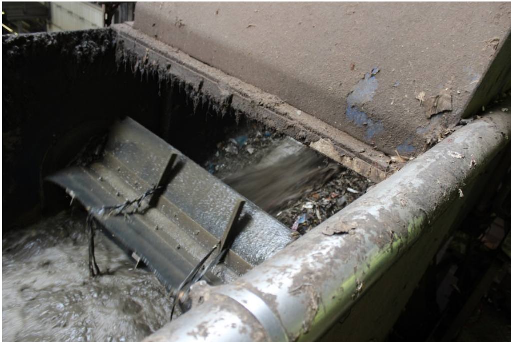
3-1-5 SBI-Omrin: Wet Organic Processing – Inert Separation
