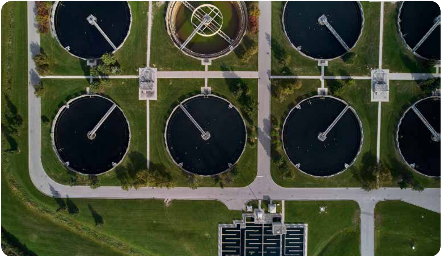
An aerial view of Duffin Creek WPCP circular clarifiers in Stage 1 and 2.
