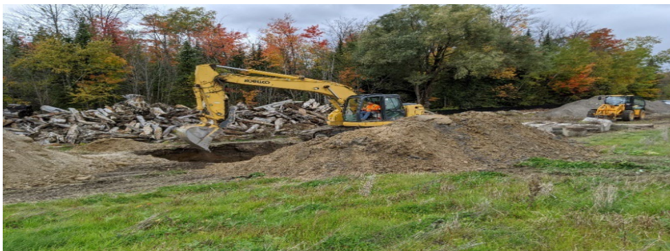
Figure: Construction of Snake hibernaculum (2020)
