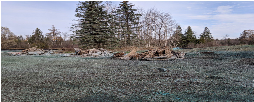
Figure: Hydro seeding and reusing logs from landfill to create habitat for small mammals (2020)
