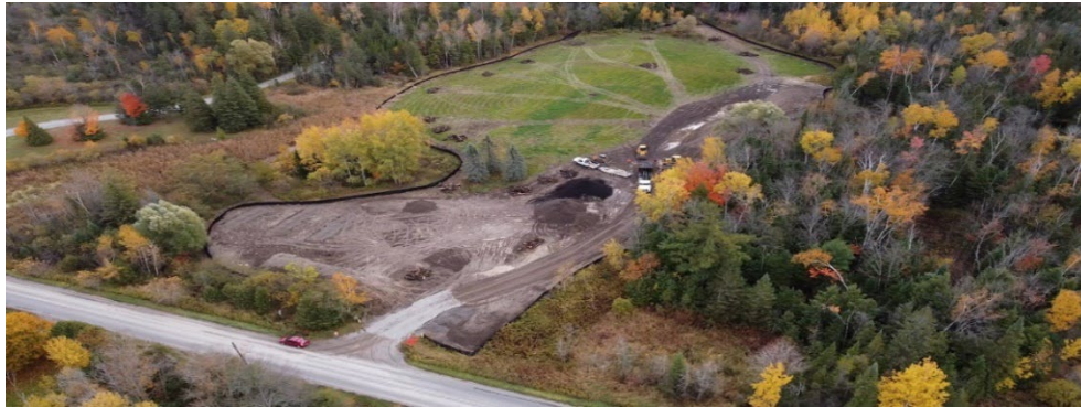
Figure: October 2020-During Construction
