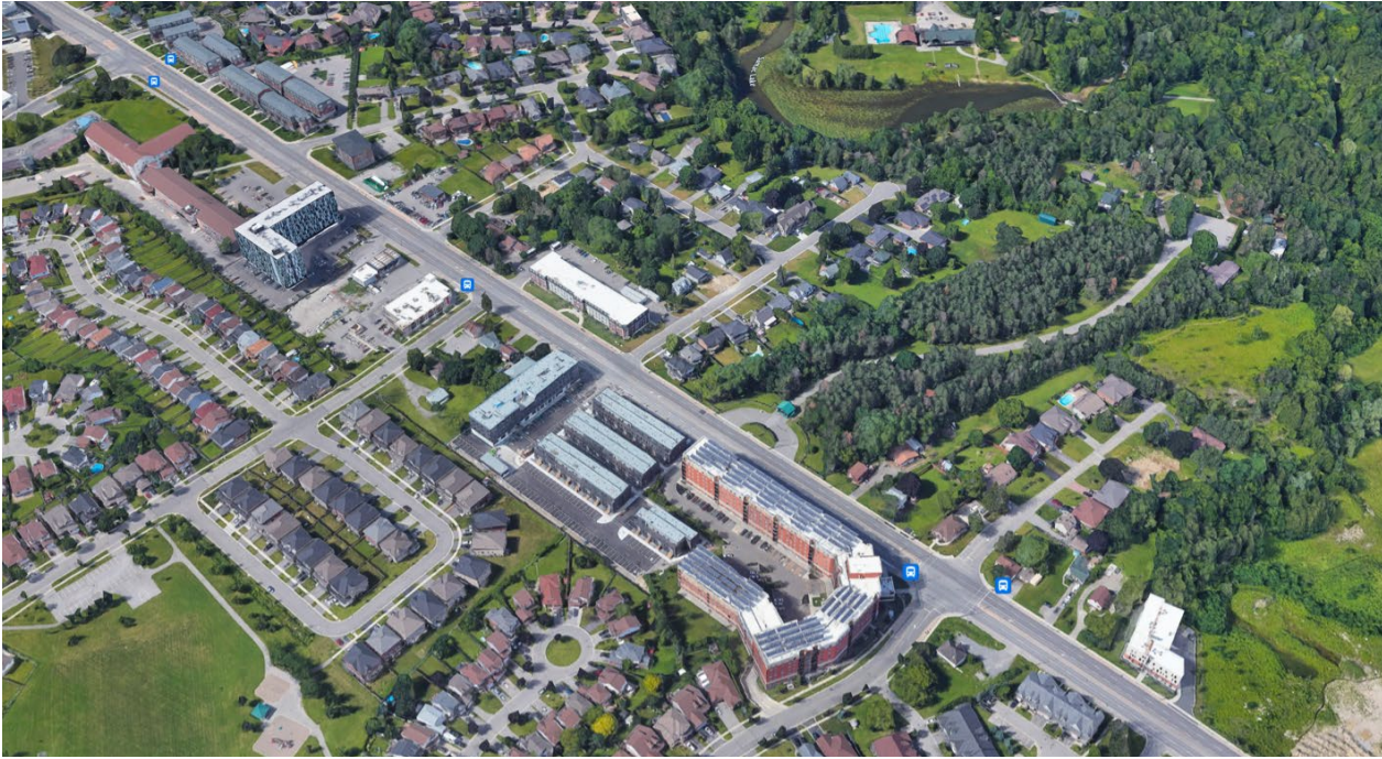
Figure 34. Oshawa (Simcoe Street North)
