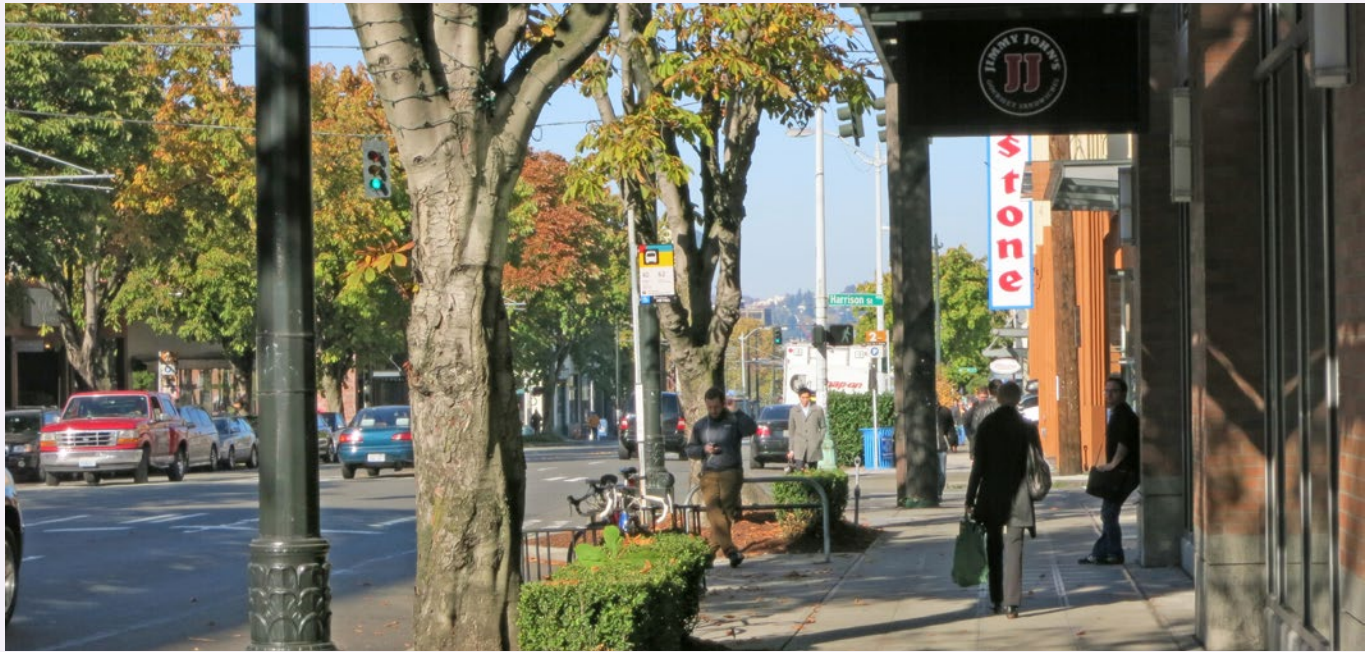
Figure 87. A large overhang provides shade and shelter for users of this bus stop.
