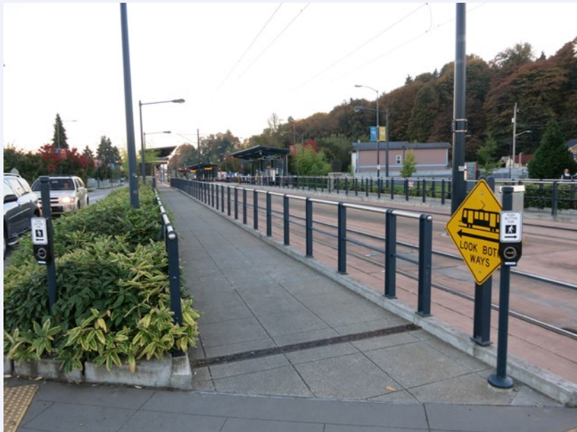
Figure 50. Safe pedestrian walkway, connecting the rapid transit corridors to stations.
