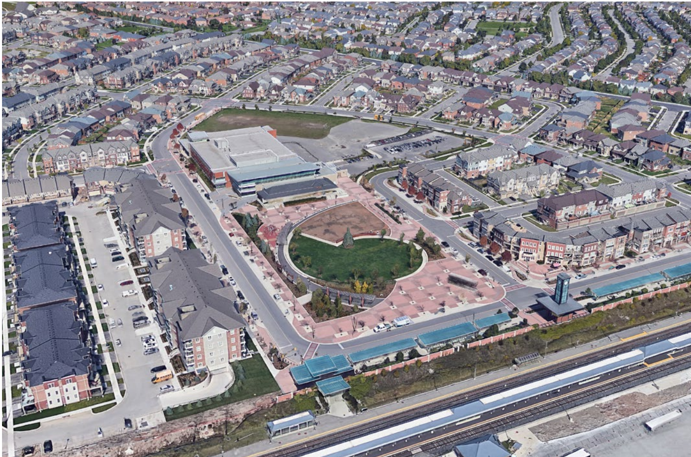
Figure 91. A transit-oriented community developed adjacent to the GO train station has been designed to extend connections to and from the station, support the station with active a mix of uses and integrate new parks and community facilities immediately adjacent to the station. Credit: Google Earth.
