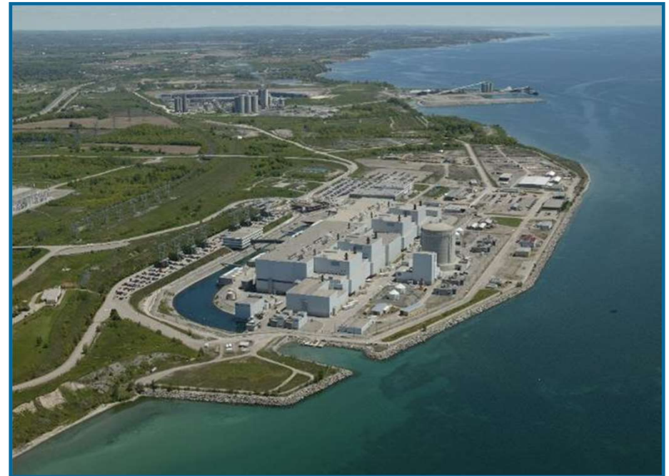
Darlington Nuclear Generating Station Source: OPG
