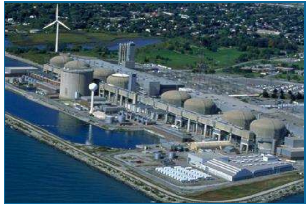
Pickering Nuclear Generating Station Source: OPG
