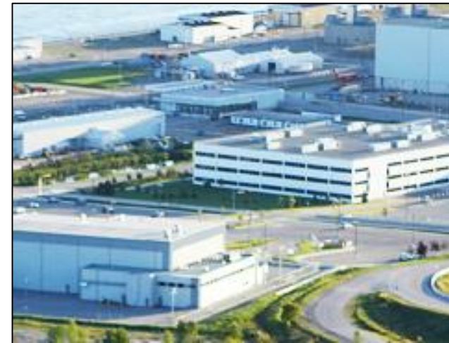
Below: DWMF, seen at lower left of photo.
