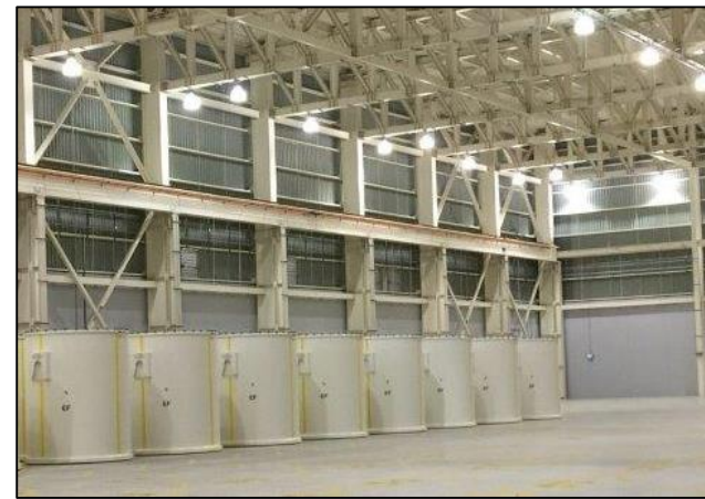
Above: Retube Waste Storage Building.
