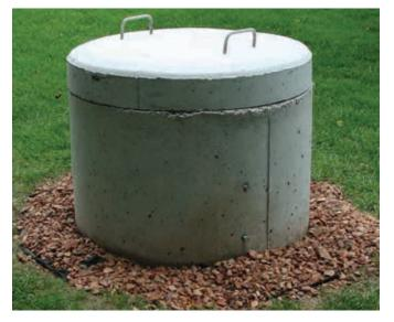
Bored wells with proper casings and sturdy well caps will help to prevent accidental falls into the well and reduce the amount of contamination that can enter the well. As with any type of well, they must be constructed and maintained properly to reduce the risk of contamination and injury.
