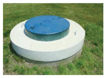
A dug well with an upgraded sturdy lid (that is properly vented and vermin proof) reduces the amount of contamination that can enter the well. Older wells of this type may have been constructed with stones, bricks, or other materials. The coloured portion of this well lid allows for observation of the well without having to removing the heavy concrete lid. The concrete lid can be removed if maintenance is required.
