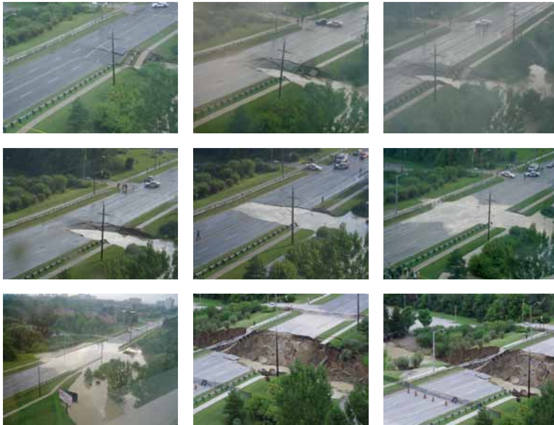
Washout of Finch Avenue in Toronto, August 19, 2005. (Photos courtesy of Jane-Finch.com)
