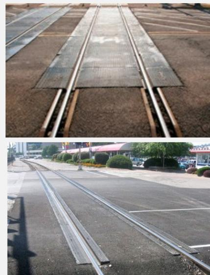
**Rubber track guards** consist of a rubber surface placed between exposed rail tracks, along an at-grade crossing. They improve the friction between tires and exposed rail along at-grade railway crossings, making it more comfortable and safer for cyclists to cross. Guards are usually accompanied by advisory signs and pavement markings.
