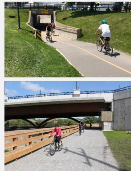
**Grade separated crossings** remove cyclists from potential conflict, by re-routing them onto new infrastructure. Structures should be designed in accordance with the MTO Structural Manual and Bridge Office Design Bulletins and Guidelines, and the Canadian Highway Bridge Design Code (CHBDC) (CAN/CSA-S6-06).
