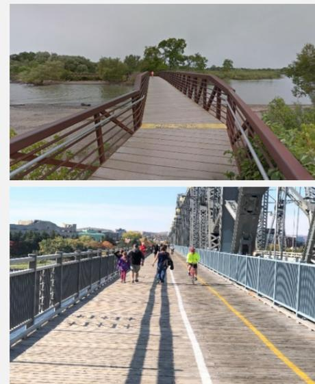
**Bridges** are separated structures built to facilitate cyclist travel over barriers imposed by natural features to improve overall network connectivity. Bi-directional cyclist bridges should feature a width of 4-4.5 metres (3.0 metre minimum while shared cyclist and pedestrian bridge should feature a width of 4-5 metres (3.6 metres minimum).
