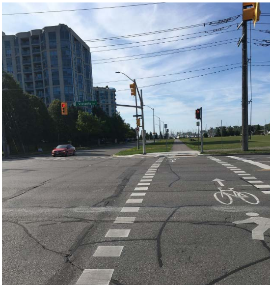
Figure 24: Cross ride at the Victoria Street/Henry Street intersection, looking south, Whitby (Source: Durham Region Planning and Economic Development Department)
