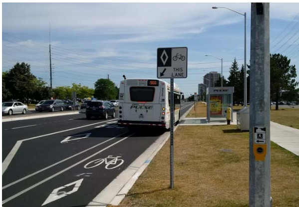
Figure 37: Recently constructed BRT and buffered bike lanes on Kingston Road, Pickering (Source: Durham Region Works Department)
