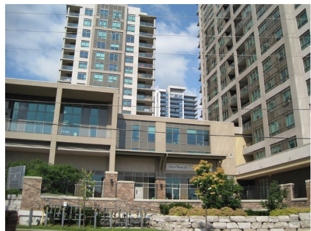
Figure 29: San Francisco by the Bay condominium development, Pickering (Source: Durham Region Planning and Economic Development Department)
