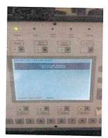
**Step #1** – Push the "Re-set" button on the Fire Panel. The LED screen will show: "LAKEVIEW MANOR – SYSTEM NORMAL" when Fire Panel has been re-set. If you do not get this message, wait approximately 10 seconds and push the "Re-set" button again.
