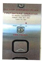
**Step #3** – Go to the elevators on 1<sup>st</sup> Floor and re-set them at the switch located directly above the heading: "FIRE RECALL"
