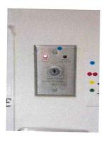
**Step #2** – Re-set the Mag-locks at the re-set switch located to the upper left of the Fire Panel. The light will indicate whether or not you have been successful.
