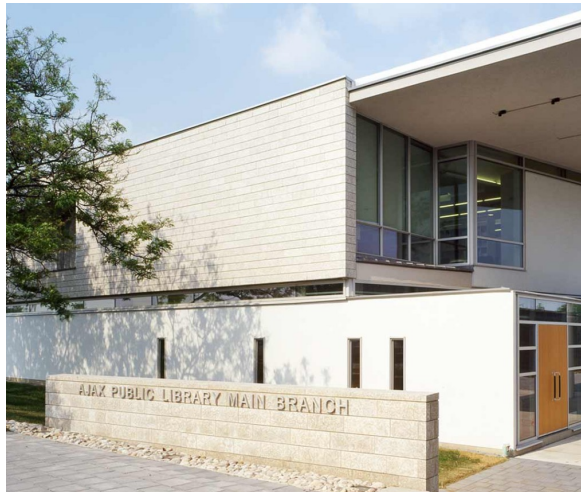
Masonry walls used at adjacent Ajax Public Library
