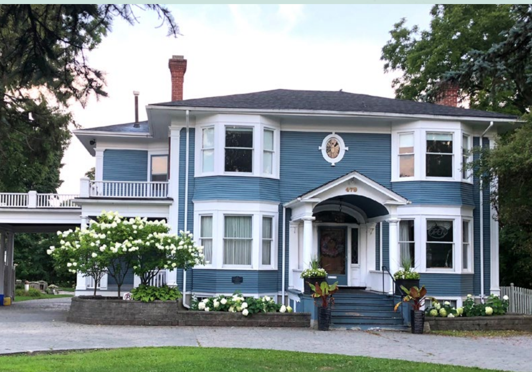
Heritage House, Pickering
