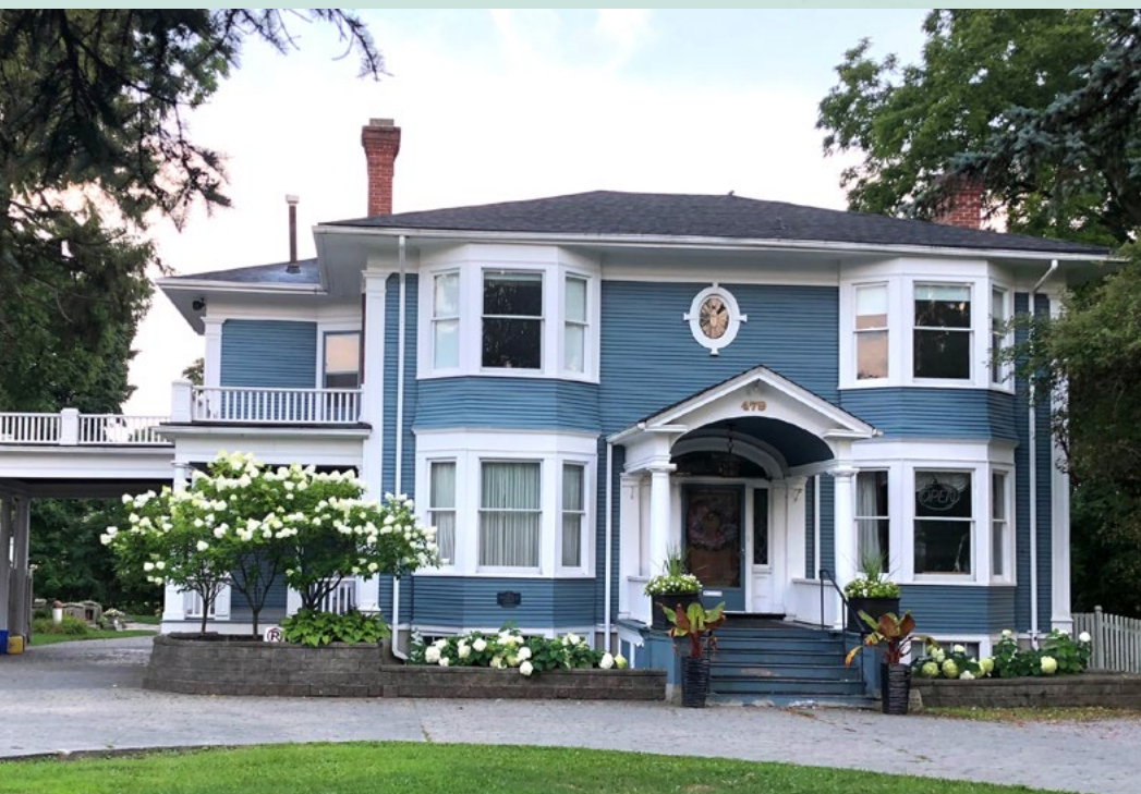
Heritage House, Pickering
